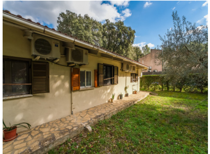
Rear view of the house
