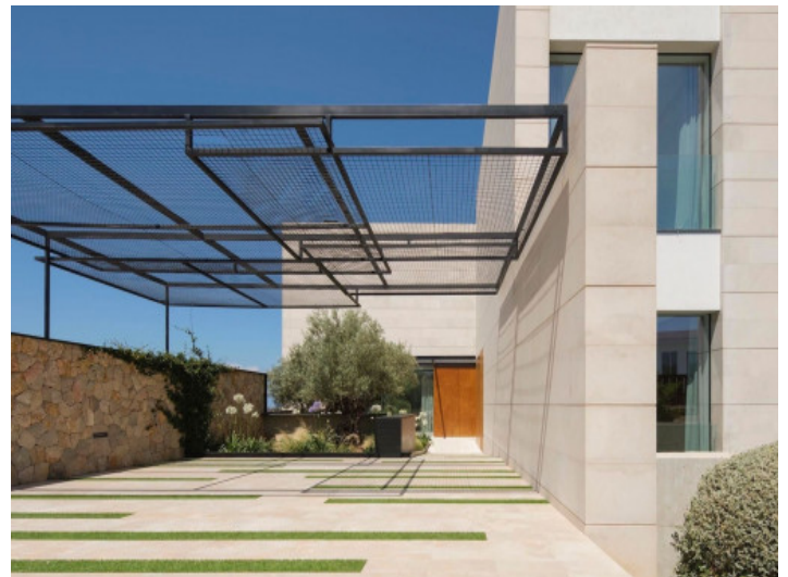
Large parking area
