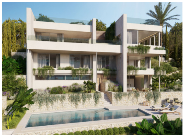
Facade and pool
