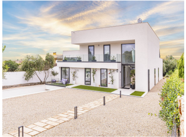
Exterior view and entrance
