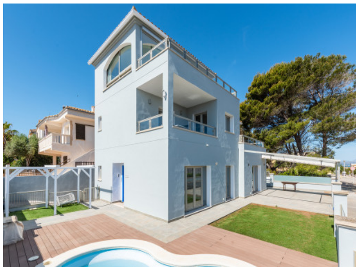
View of the house
