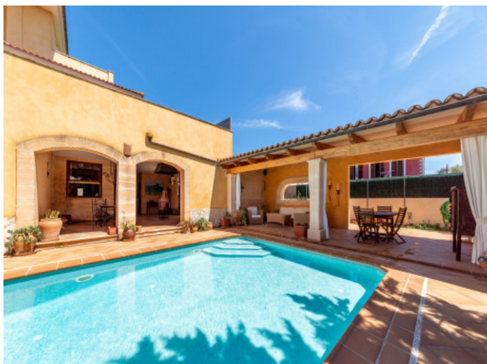
Pool area and covered terrace
