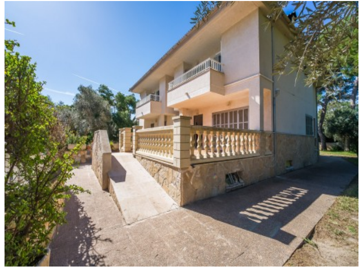
Sunny terraces and balconies
