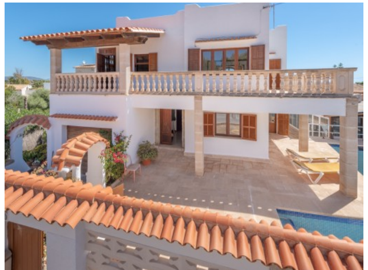
Front view and entrance to the house
