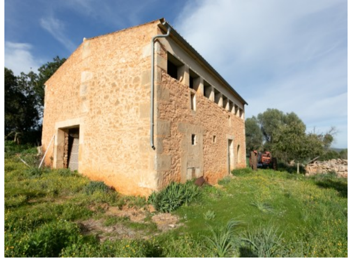
A 2-storey house already exists
