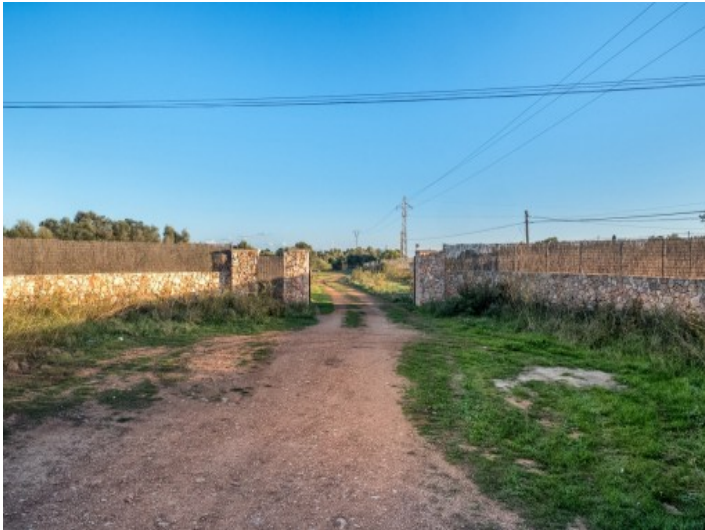
Views of the wall
