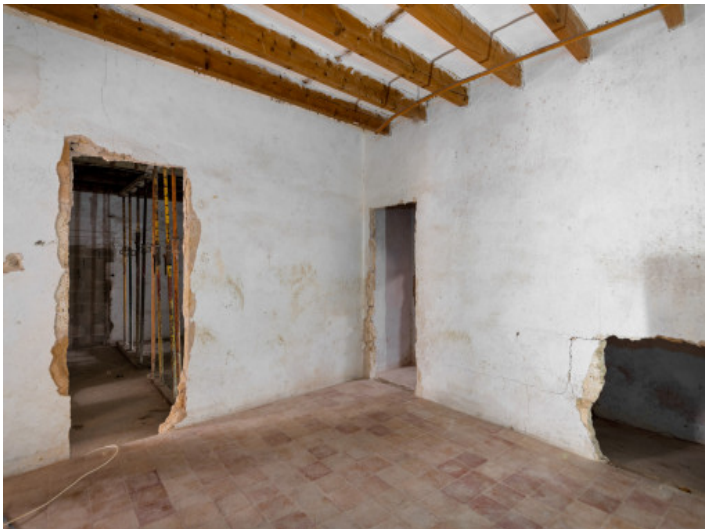
Old wooden beams
