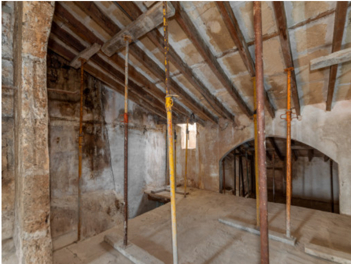
Original wooden beams
