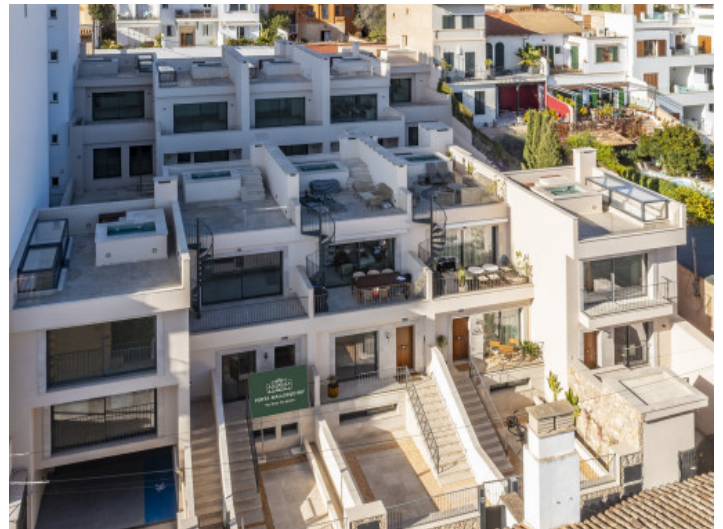
Terraced house with 3 levels and rooftop
