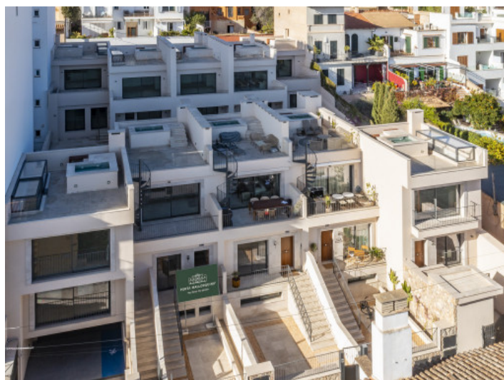
Terraced house with 3 levels and rooftop
