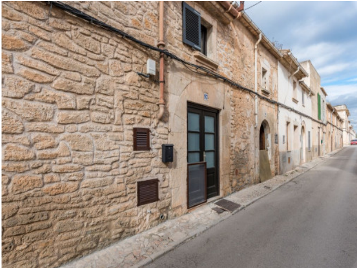
Exterior view of the town house
