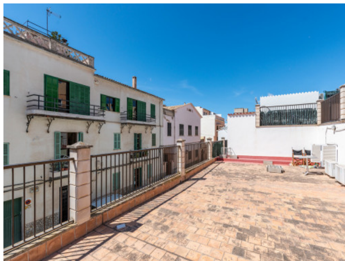
Lower part of the roof terrace
