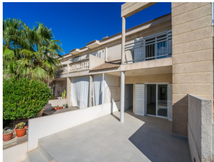
Front terrace and access to the house
