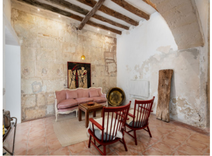
Restored sandstone walls
