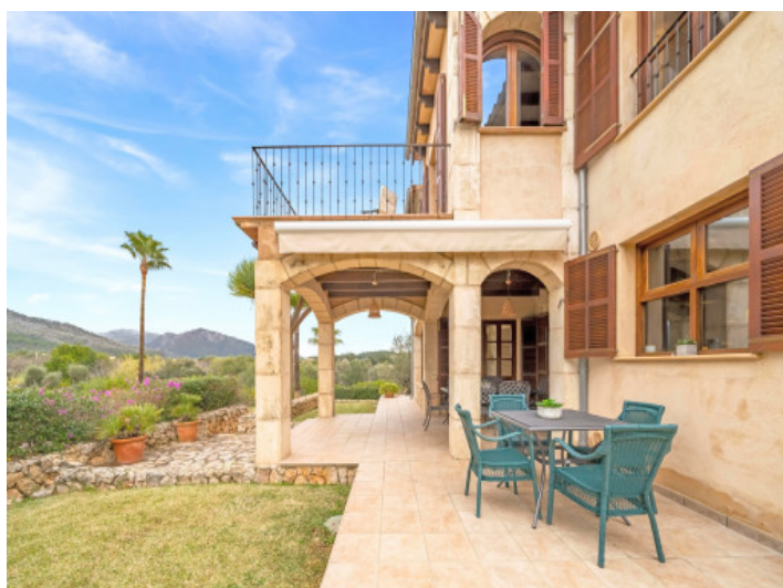
Natural stone facade
