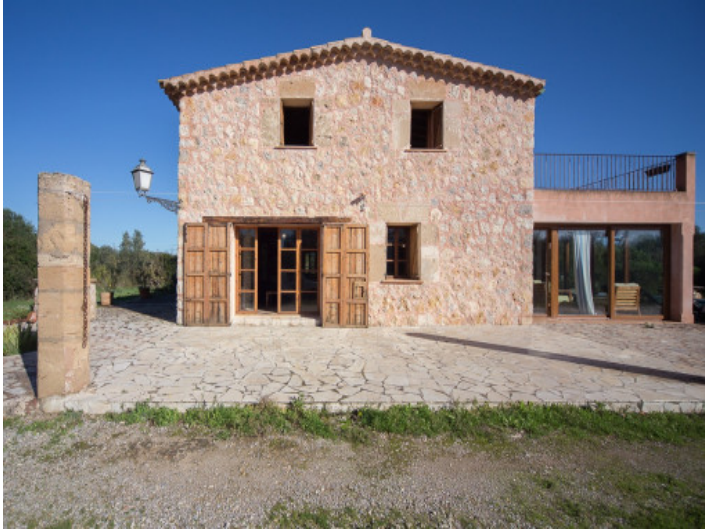
Traditional stone-clad façade
