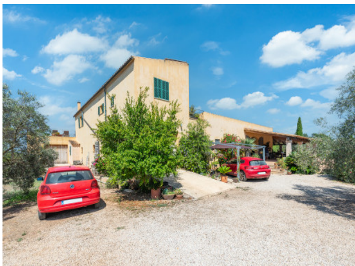
Access to the house
