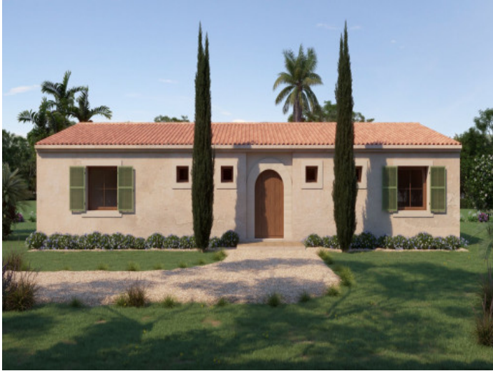
Exterior and entrance area
