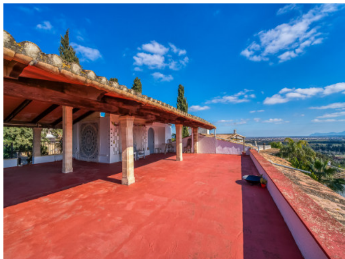
Extensive roof top terrace
