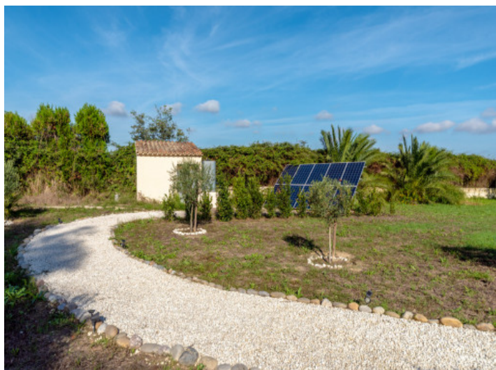
Plot with solar panel
