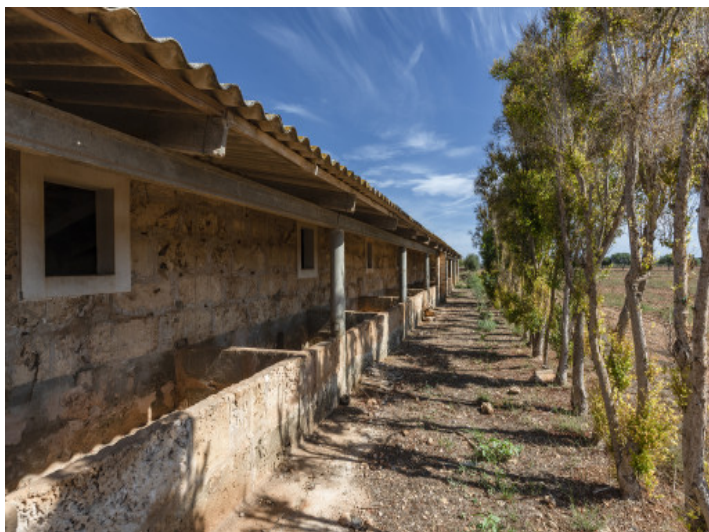
Exterior view of the property
