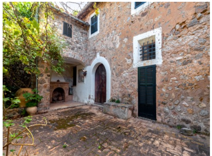
View of the natural stone facade
