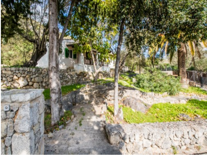
Access to a guest house
