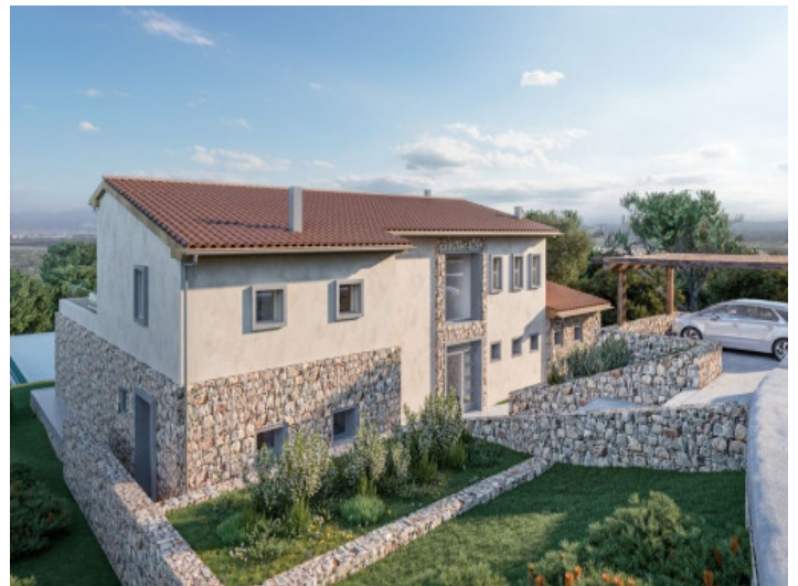
Exterior view and access
