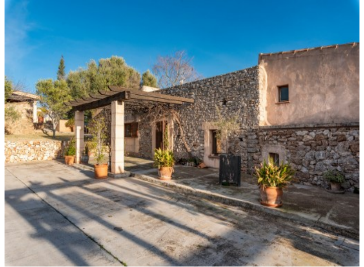
Front view and access to the house
