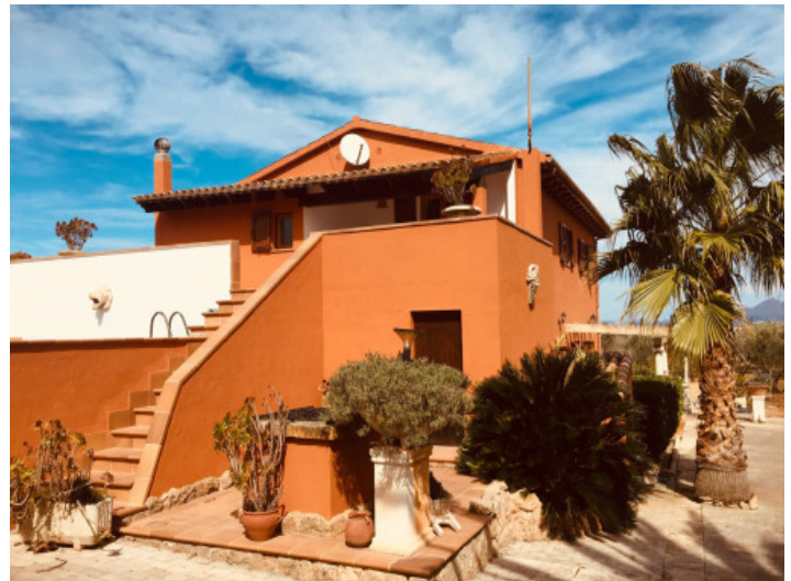
View from the south
