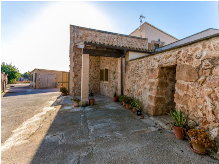
Typical natural stone walls
