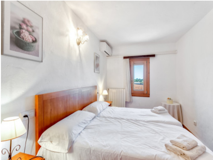
Air conditioning and heating in the bedroom
