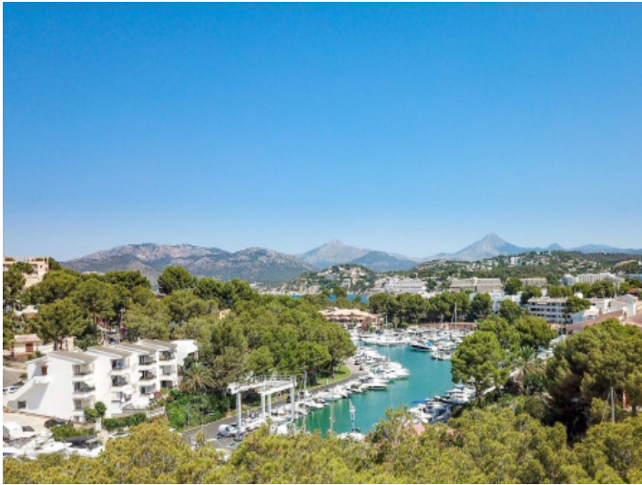
Villa construction project with harbour views in Santa Ponsa
