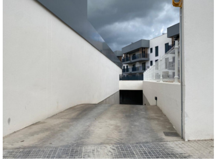
Access to the underground parking
