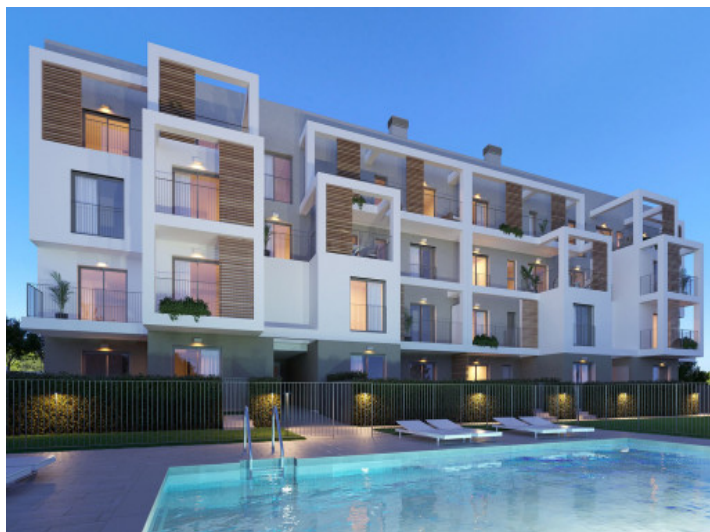
View to the building
