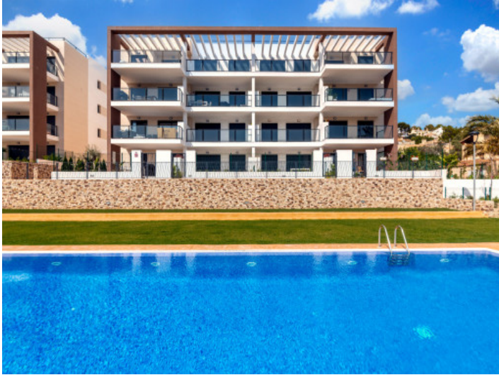
Complex and pool
