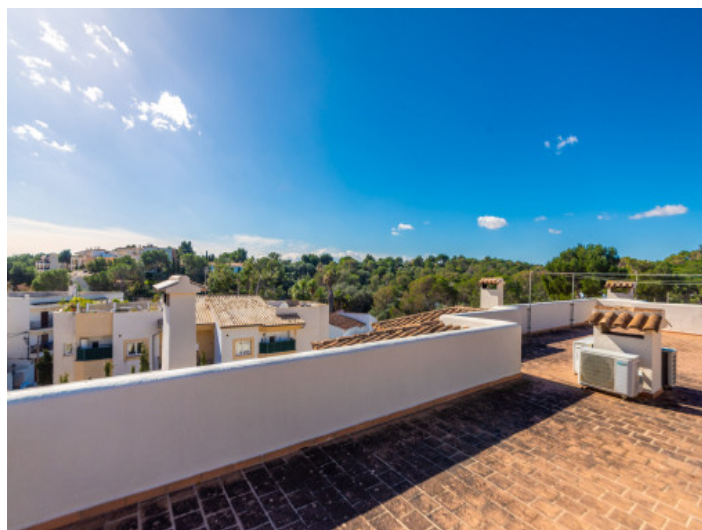
Roof terrace of the building
