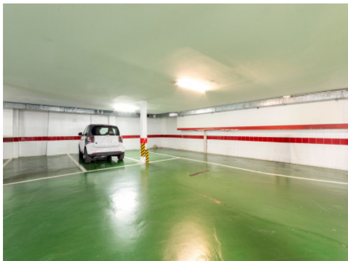
Underground parking space
