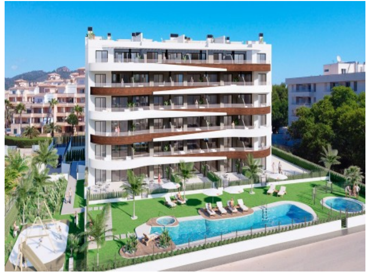
Complex and pool
