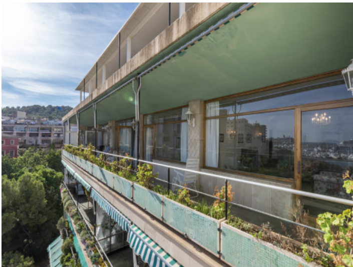
Exterior or balcony view
