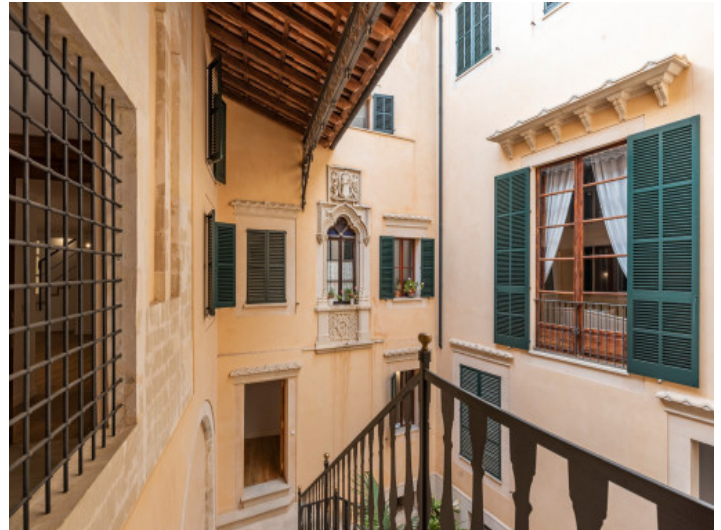
Access to the patio
