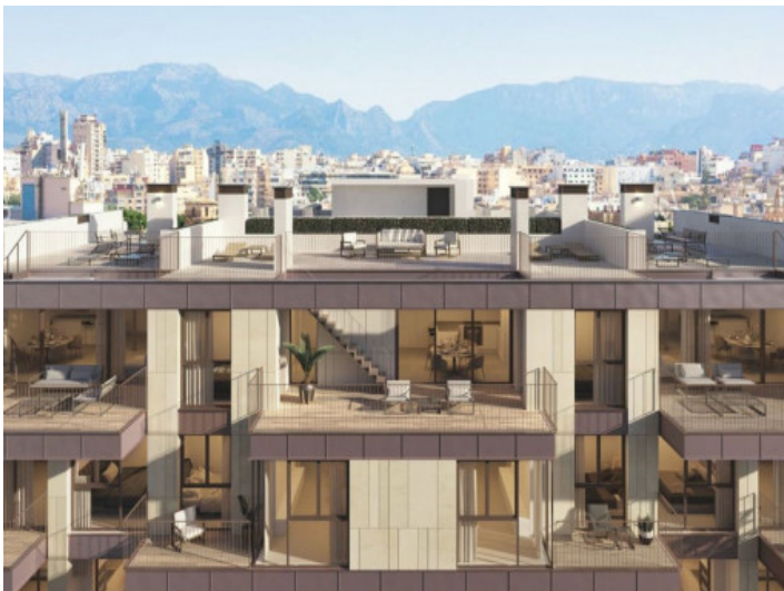
Front view of the residential complex
