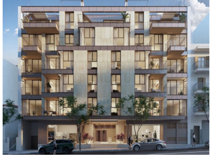
Front view of the residential complex
