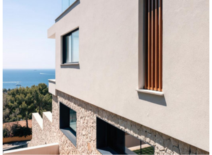
Lateral facade and views
