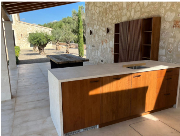
Covered terrace with summer kitchen
